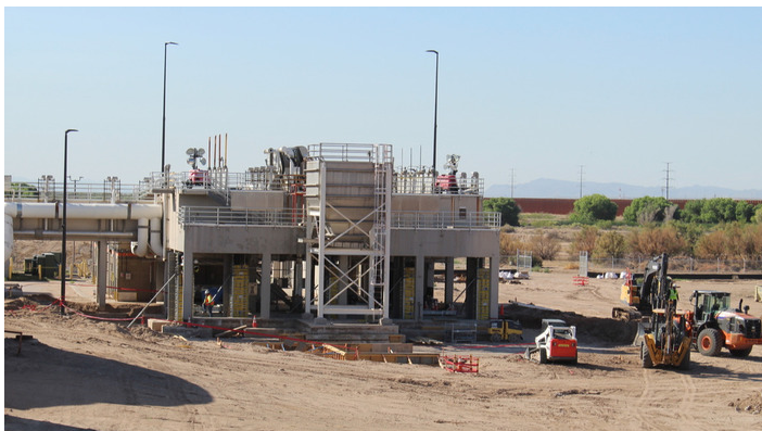
Construction is taking place at the Bustamante Plant.
